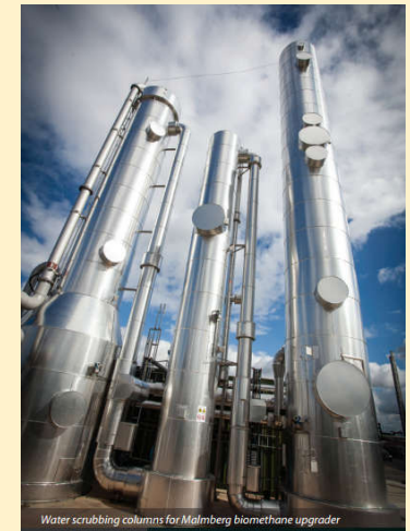
Water scrubbing columns for Malmberg biomethane upgrader
