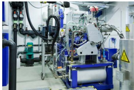
Engine test bed
