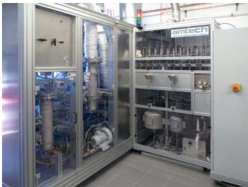
Fuel technical centre
