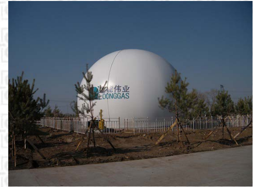
双膜储气柜 Biogas tank
