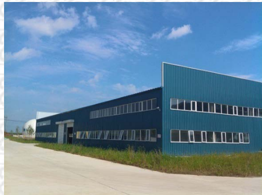
处理车间 Treatment plant
